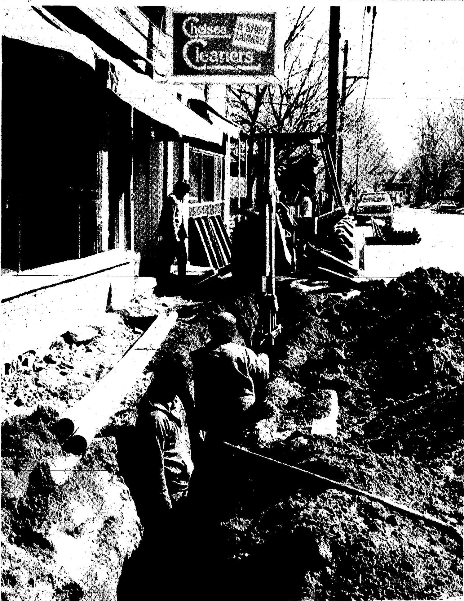
MICHIGAN BELL has been tearing up Park St. sidewalks in order to install new underground telephone lines. The project will also continue under sidewalk down
